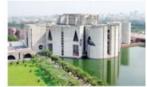
National Assembly Building “LOUIS- I KAHN”
