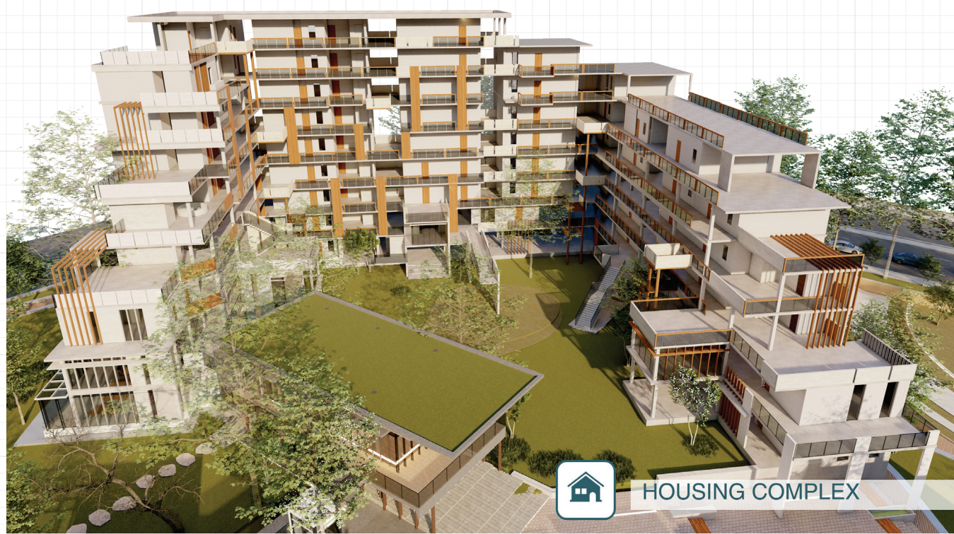
Fig 64. View Towards the Courtyard of the Housing Block
